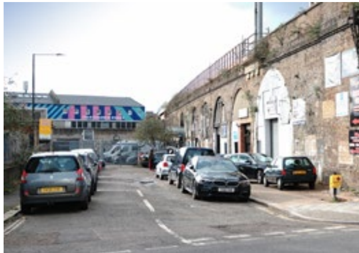
Railway arches on Hardess Street
